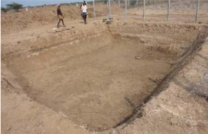
Figure 7: Percolation pond construction in Andarmadam
