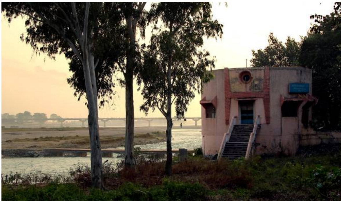
Figure 2-3 Example of large-diameter RBF well adjacent to Ganga River, Haridwar (Photo: L. Rossoff, HTWD, 2011)
