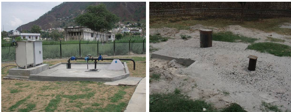
Figure 8-1 Sanitary sealing of production wells PW-DST (left) and PW5 and MW5 (right) at Srinagar RBF sites implemented by UJS (photos: Heinze and Lesch 2012)
