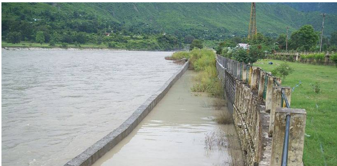
Figure 3-2 View of flood-wall (left) and retaining wall (right) of the lower level of the park where the RBF site in Srinagar is located (Photo: M. Ronghang, IITR, 2011)
