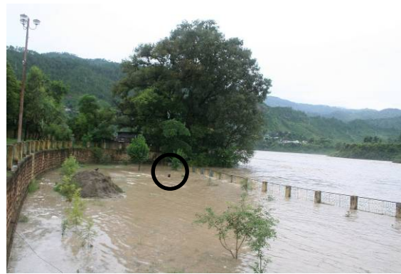
Figure 2-10 Production well PW5 (under construction) in the background (encircled) inundated by the monsoon flood of the Alaknanda (facing downstream) in August 2011 (Photo: J. Ebermann, HTWD, 2011)
